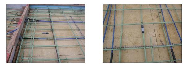
Figure 4: Use of Tags in Slab Pour in Mid-slab Portion and at edge of Slab (Courtesy PSI Inc.)
