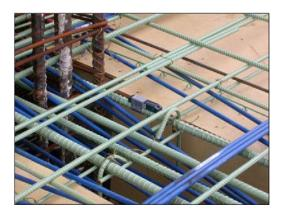
Figure 5: Use of Tags in Beam Pour Troughs amidst the Tensioning Strands (Courtesy PSI Inc.)
