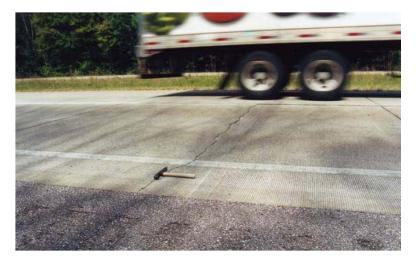
Figure 17: Photo showing Premature Cracking due to negative temperature gradients (University of Michigan, Ann Arbor)
