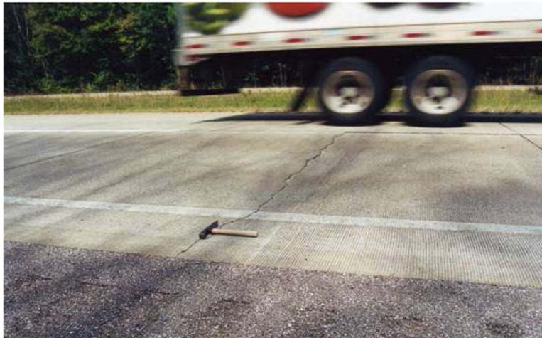
**Figure 17:** Photo showing Premature Cracking due to negative temperature gradients
