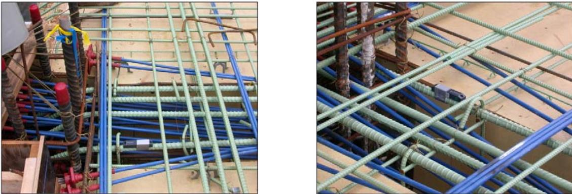
**Figure 5:** Use of Tags in Beam Pour Troughs amidst the Tensioning Strands (Courtesy PSI Inc.)
