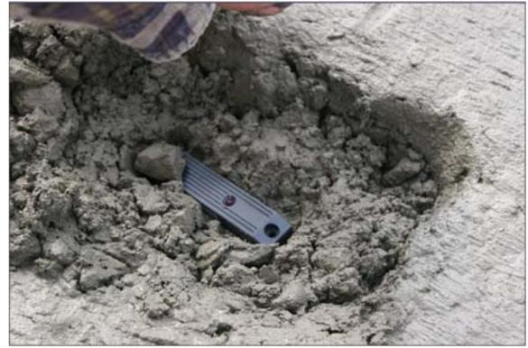
**Figure 10:** Scooping out of fresh concrete and placement of tags (University of Michigan, Ann Arbor)
