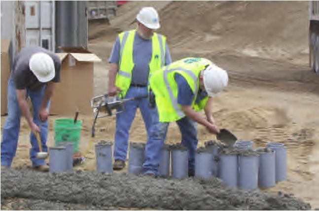
Construction crew making Test Cylinders
